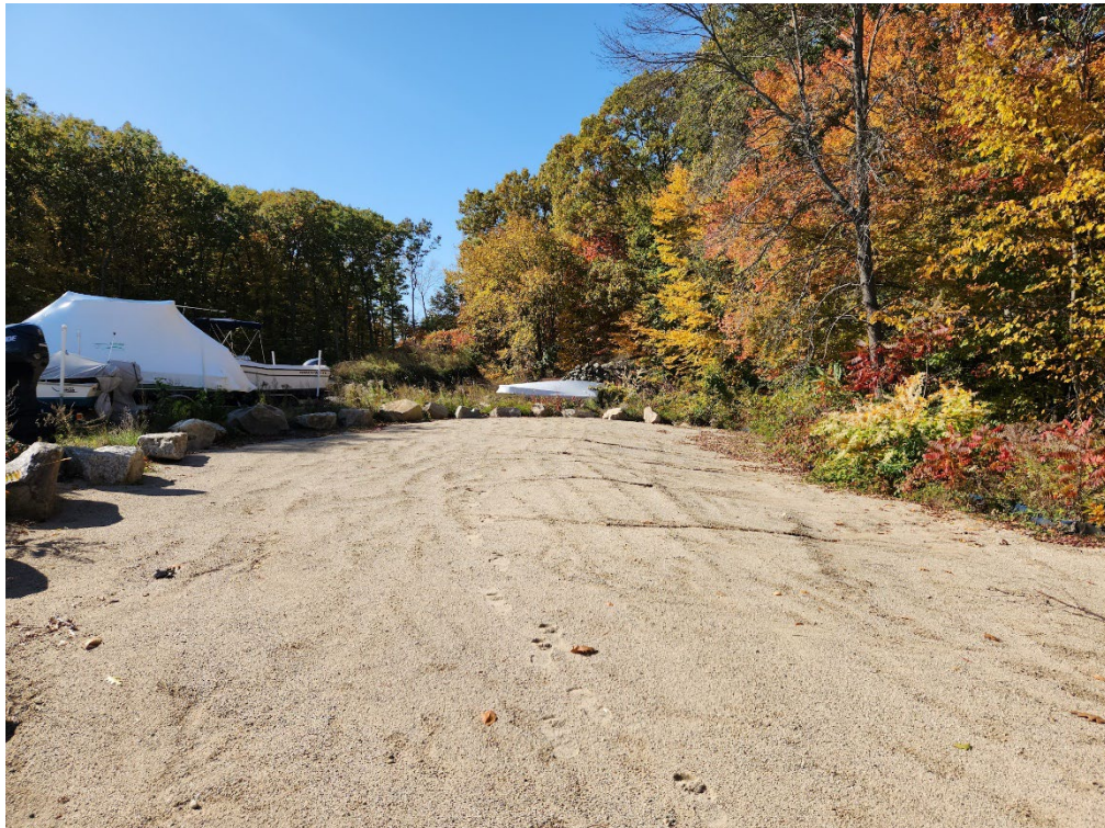
Photo 13: October 2022 - PCB excavation area covered with sand and marker barrier.
